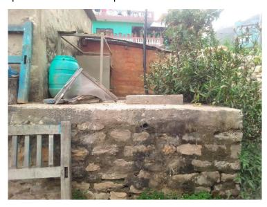
Figure 6: Lined tank with impermeable walls and open bottom in the Shaarada Municipality.
